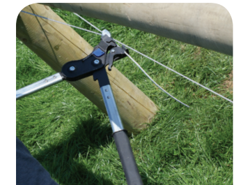
Apply tension with a Contractor Tool
