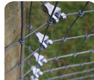
Terminate at an end-post with Gripple T-Clip
